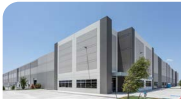
MESQUITE AIRPORT LOGISTICS CENTER
