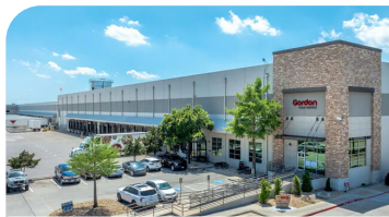
FREPORT CROSSING BUILDING 4
